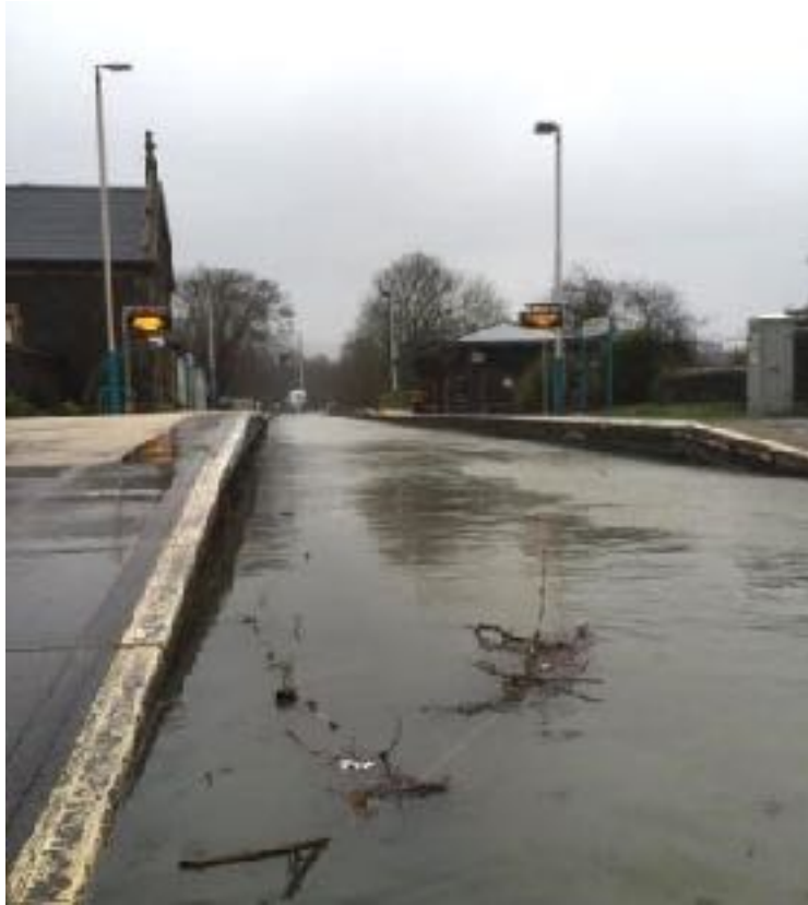
Flooding at North Llanrwst station, North Wales - January 2016
