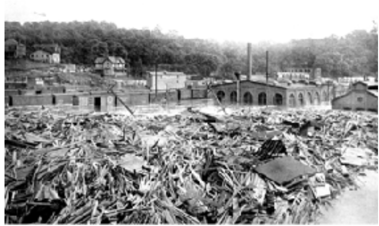
Seriously, flooding can bring destruction. The piles of timber brought down by the flooding in Asheville, North Carolina, July 1916 following the destruction of buildings, mills, homes and many businesses.
